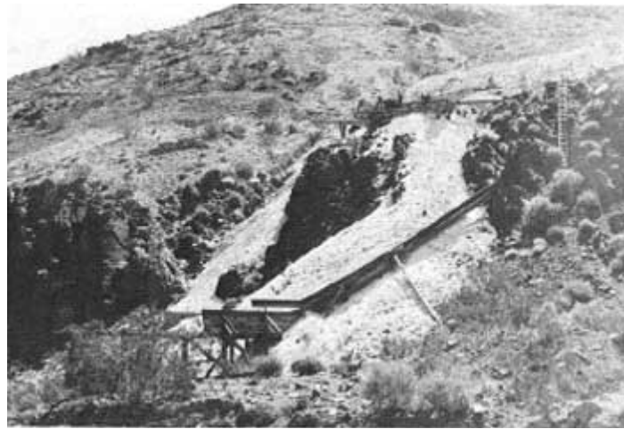
Illustration 66. Claim immediately east of Warm Spring Camp in Warm Spring Canyon (#8 on site map). Possibly Old Quartz Millsite Claim or Old Mill Stream Claim? Photo by Linda W. Greene, 1978.
