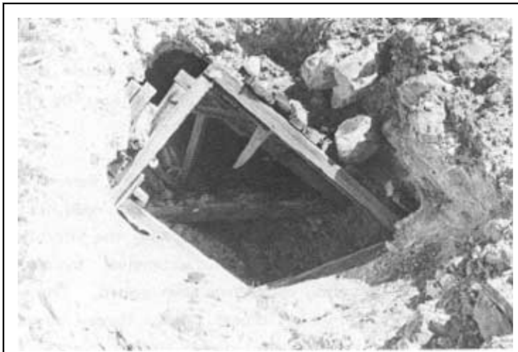
Illustration 59. Timbered adit (#1 on site map) north of Warm Spring Canyon Road. Photo by Linda W. Greene, 1978.
